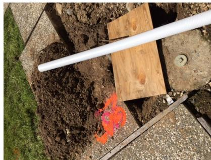
Although functioning properly at the moment, both buildings need additional plumbing attention. The Preschool building needs an extra clean out installed and the Rectory needs 10' of pipe dug up and replaced to remedy the current problems.
