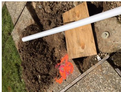
Although functioning properly at the moment, both buildings need additional plumbing attention. The Preschool building needs an extra clean out installed and the Rectory needs 10' of pipe dug up and replaced to remedy the current problems.
